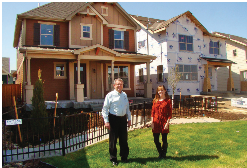
Wonderland Vice President Michael Hart and Amy Irvin show one of the traditionally styled Heritage models opening this weekend at Stapleton's Conservatory Green neighborhood.
