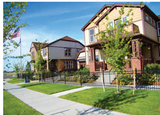
The builder, with some of their last homes in Stapleton's Central Park West neighborhood, is readying a choice selection for summer move-in.
